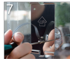
7 Slide the bracket to the left and tighten the bolts.
